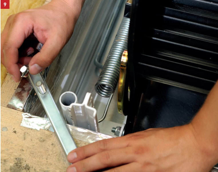
Fastening the frame using the 4 supports
