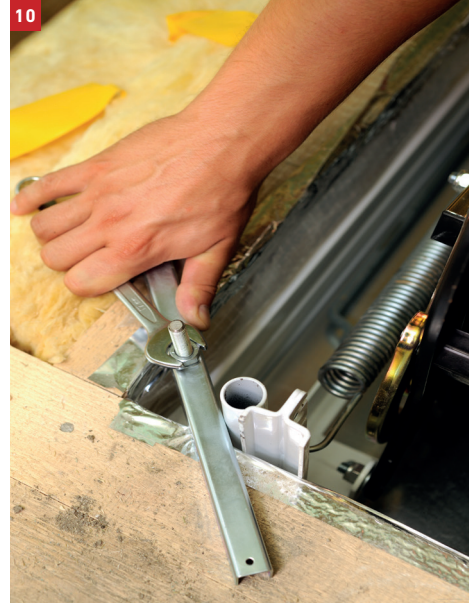
Proper fastening of the 4 anchoring bolts
